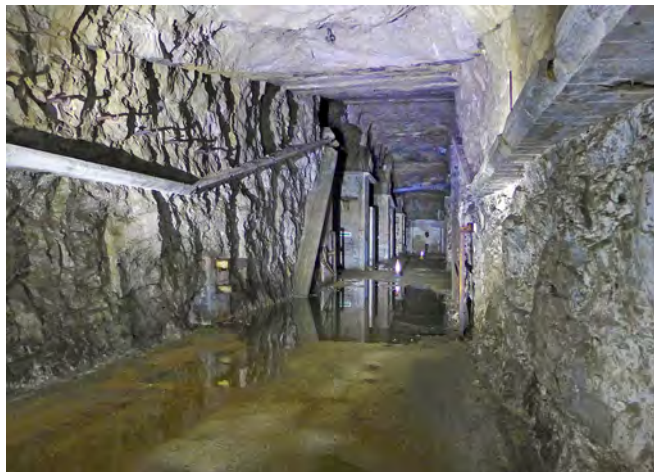
Looking west along the central tunnel just before the junction with chamber 'A', the entrance is behind the photographer. Note the slope showing the ventilation arrangement. The incoming fresh air would have been directed above a false ceiling and extracted from below floor-level
